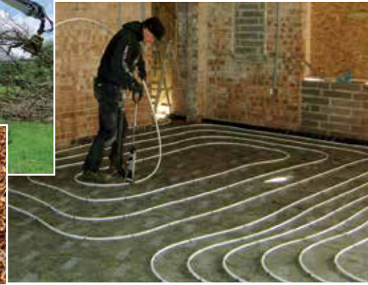
The heat is fed through an under floor thermostatically zoned system.
