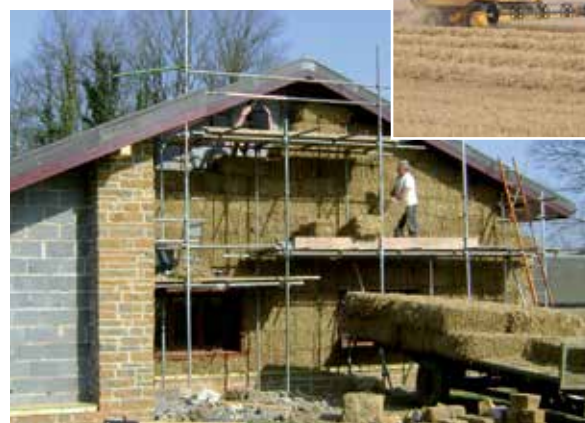
The wall insulation is constructed of straw bales made from the farm's own wheat straw.
