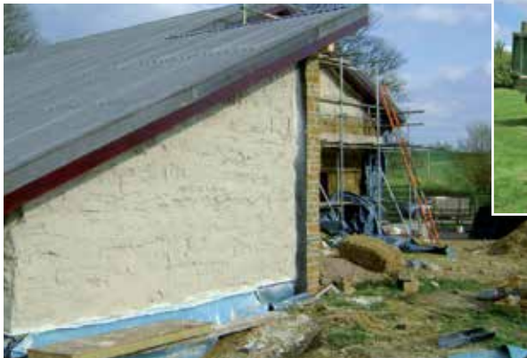
The straw bales are rendered with lime mortar.
