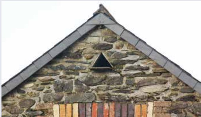
An entrance for barn owls built into a barn converted for holiday lets
