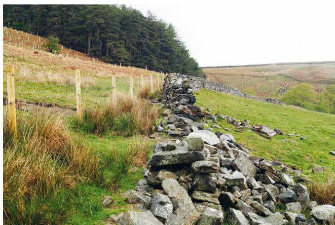
1,200m of walls are being repaired and 64,000 trees planted.
